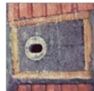
On-site insulation to avoid thermal bridges
