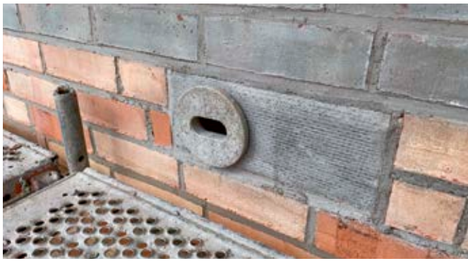
▲ Fig. 3: Installation in the brickwork
