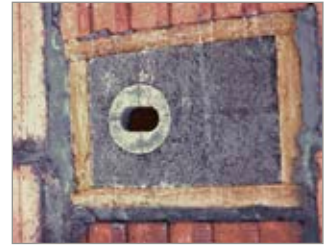
▲ on-site insulation to avoid thermal bridges
